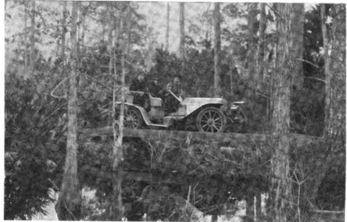
CROSSING ONE OF THOMAS WHITE'S TRESTLES.
